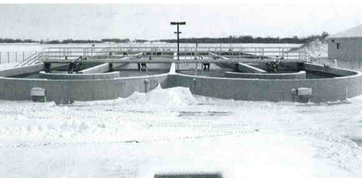
A view from the west end of the two-ring oxidation ditch at Dawson, MN. The DO probes are mounted in the foreground in the corner of each ditch near the center dividing wall.
